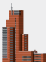
Wintower, Winterthur 1999, 90 m
